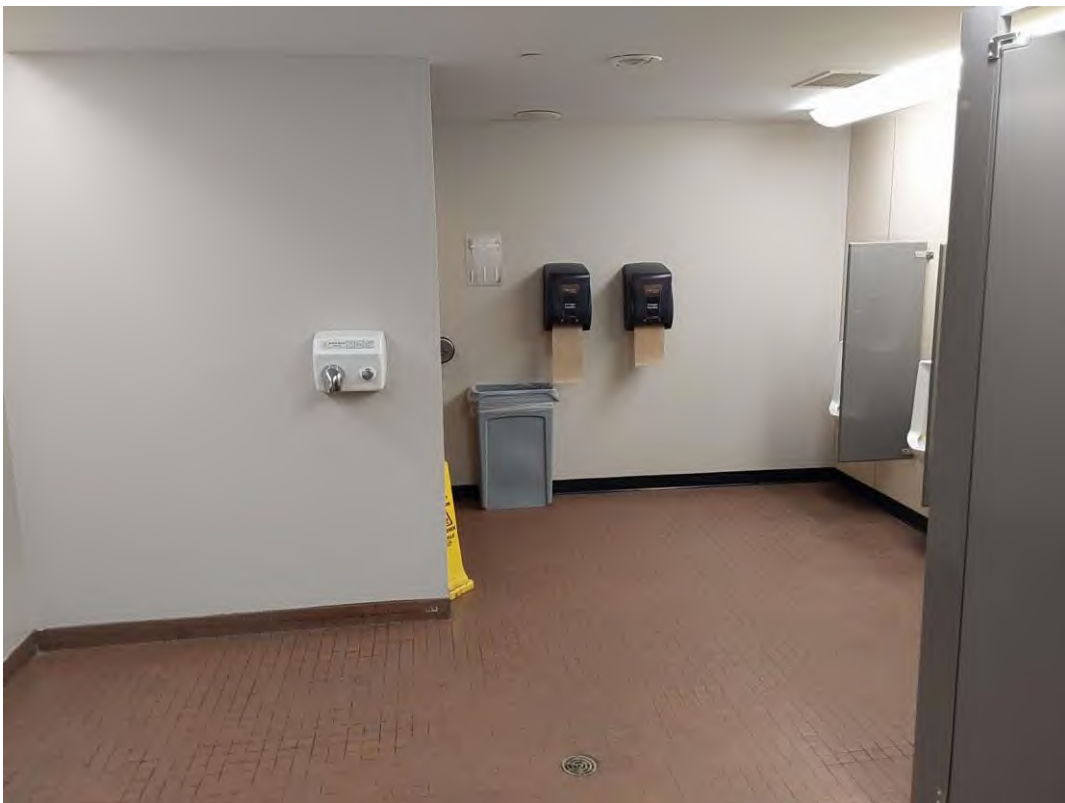
Men's Washroom - B3174 (Location #: 191)
