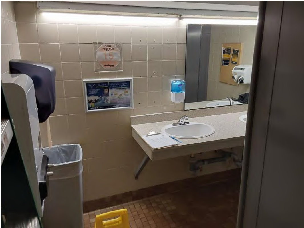
Women's Washroom - C2128 (Location #: 404)
