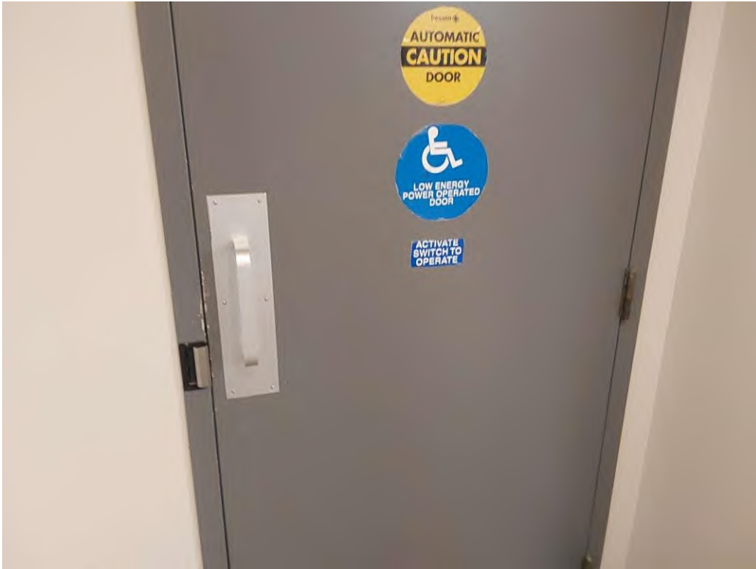
L0008(Lead, Low), Grey paint on door, Wall, Men's Washroom - B3174 (Location #: 191)
