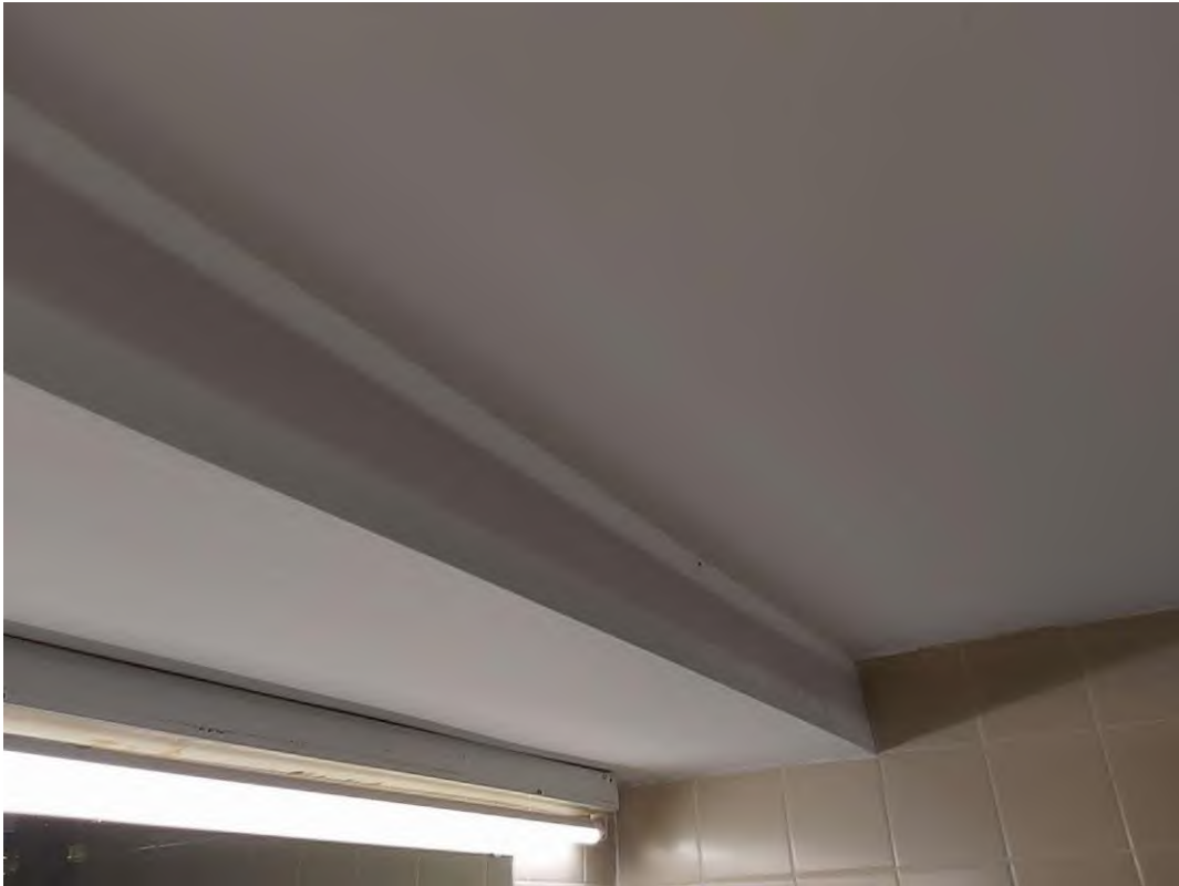
S0076C (None), Ceiling, Drywall and joint compound, Men's Washroom - C2126 (Location #: 403)
