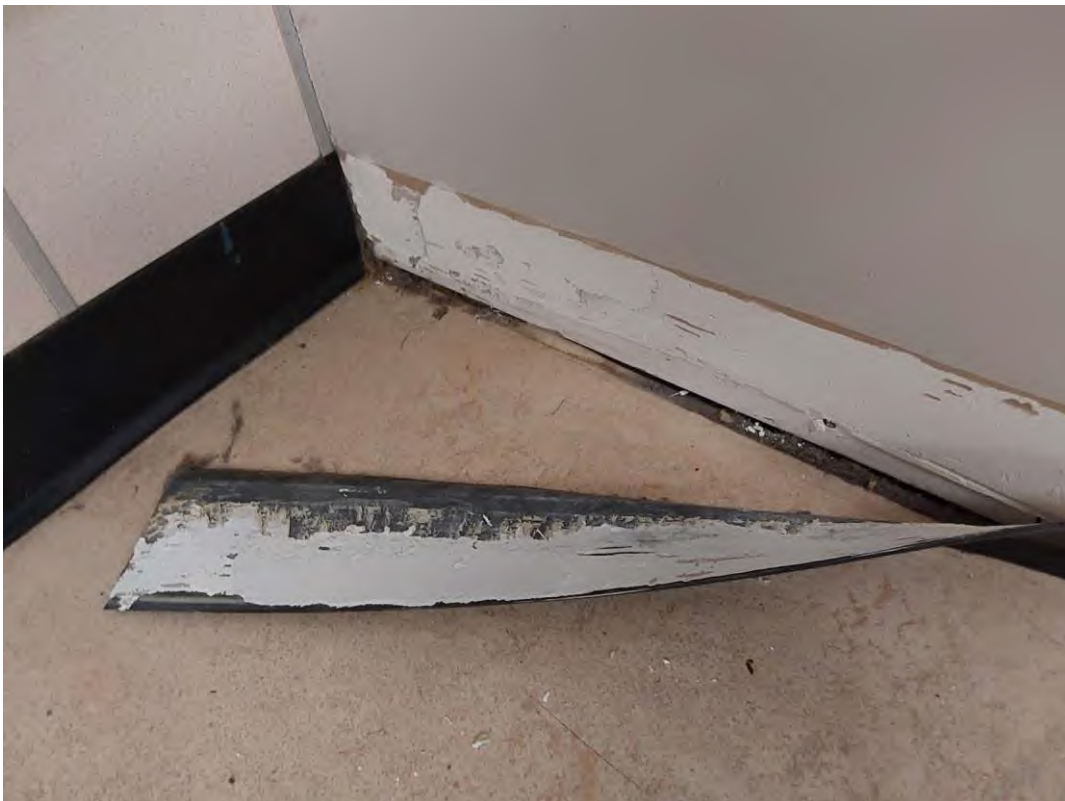
S0080C (None), Beige baseboard mastic, Wall, Adhesive/mastic, Women's Washroom - B3170 (Location #: 190)
