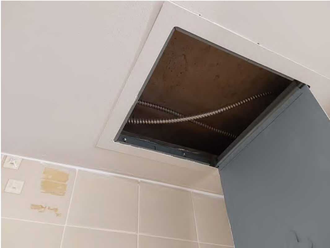
Structure, Concrete (poured), Men's Washroom - C2126 (Location #: 403)
