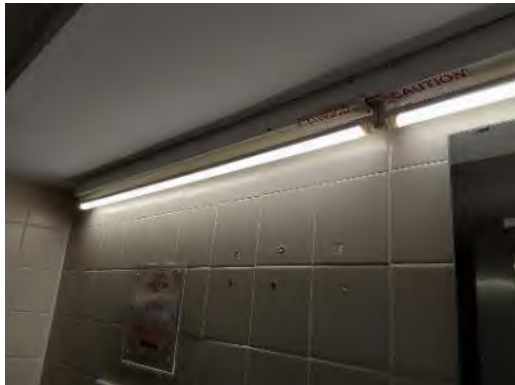
Light Emitting Diode (LED) T8 lamps in the Men's Washroom - C2126 (Loc. 403)
