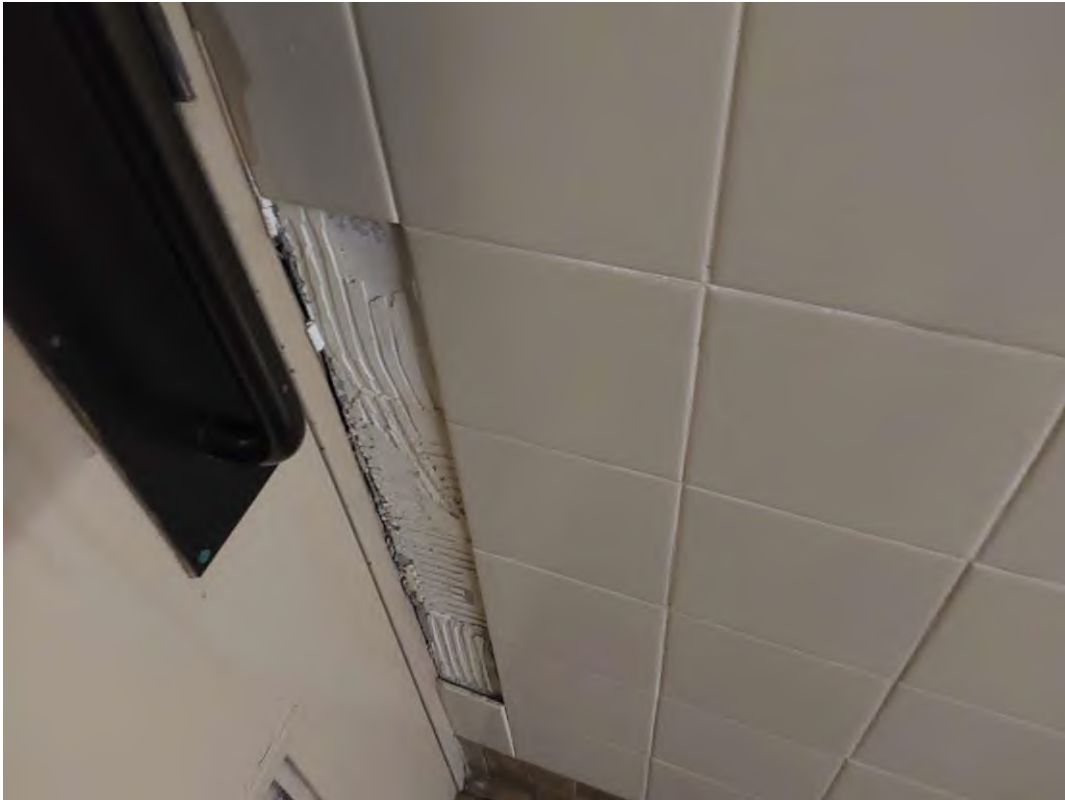
S0073A (None), Wall, Mortar, Women's Washroom - C2128 (Location #: 404)
