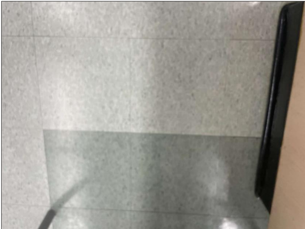
V0000 (None), 12x12 mottled light blue, Floor, All, Vinyl Floor Tile and Mastic, 238 (Location #: 2820) Previous samples ASB-111.1-3
