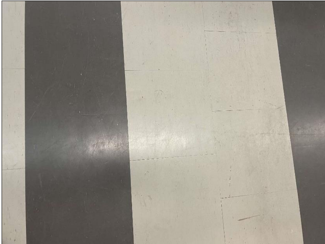
V9000 (Confirmed Asbestos), VT-9, 12x12, off-white, Floor, Vinyl Floor Tile, 233 (Location #: 2310) Historic data
