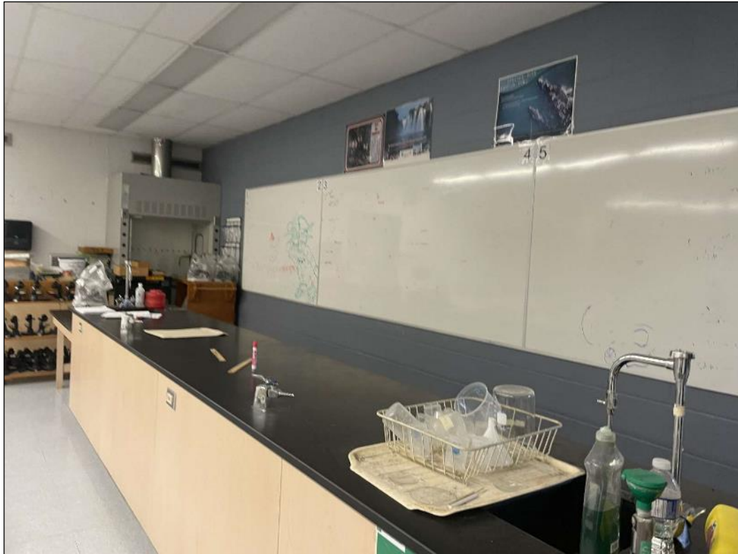
V9500 (Presumed Asbestos), Other, Countertop, Cement Product, 238 (Location #: 2820)
