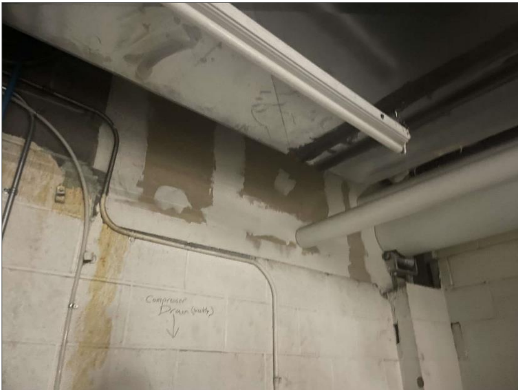
S0015A (None), Wall, Paint, 300 (Location #: 301)
