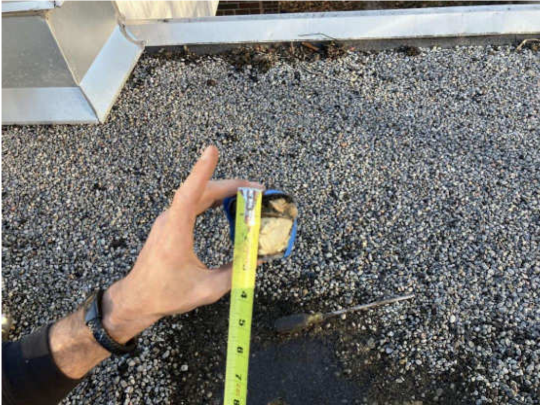
S1019A (Non-asbestos), Roofing materials, Roof E (Location #: 214)
