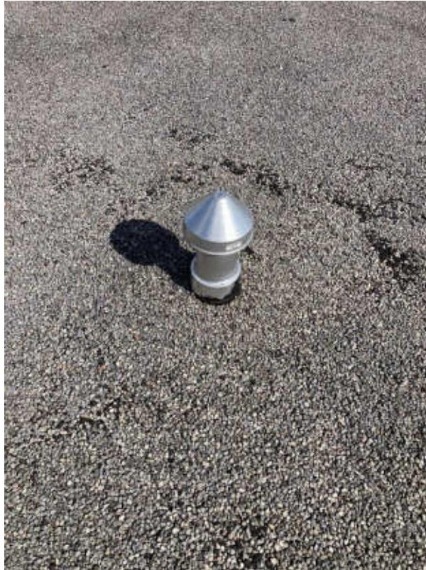
S1016A (Non-asbestos), Black tar on vent, Roof B (Location #: 210)
