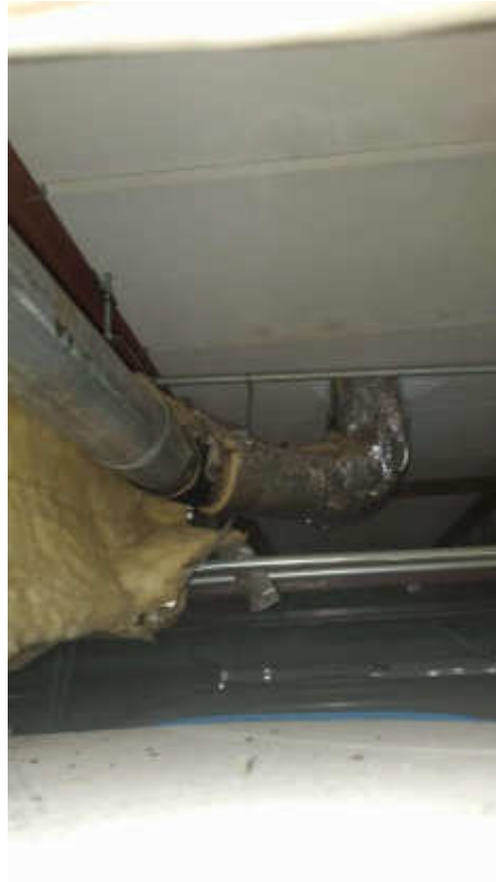
Piping, (non-asbestos) Fibreglass insulation on Rainwater Leader, Staff Room (Location #: 190)
