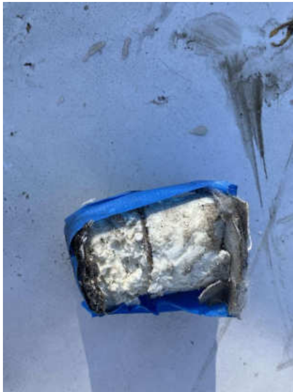
S1018A (Non-asbestos), Roofing materials, Roof D (Location #: 213)
