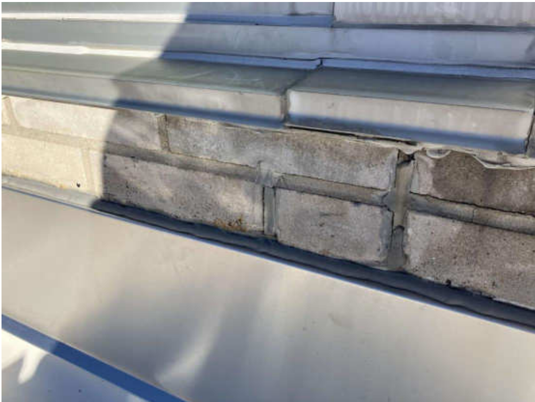
S1020A (Non-asbestos), Grey caulking on flashing, Roof D (Location #: 213)
